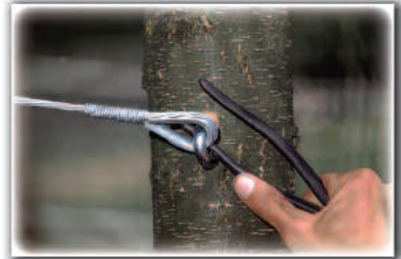
Cabling adds strength to trees, helping them to stand up to snow, ice and wind damage.
